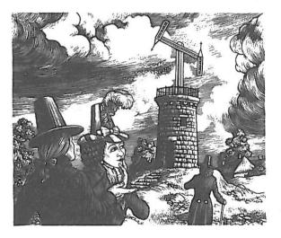
Operators in each tower watched neighbouring towers through a telescope and then passed the message on to the next one in the line. The first line stretched from Paris to Lille, a distance of 230 km.
